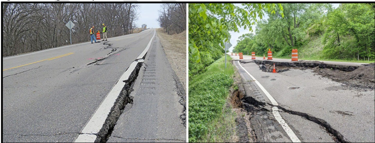
Hwy 67 failure due to unstable ground.
