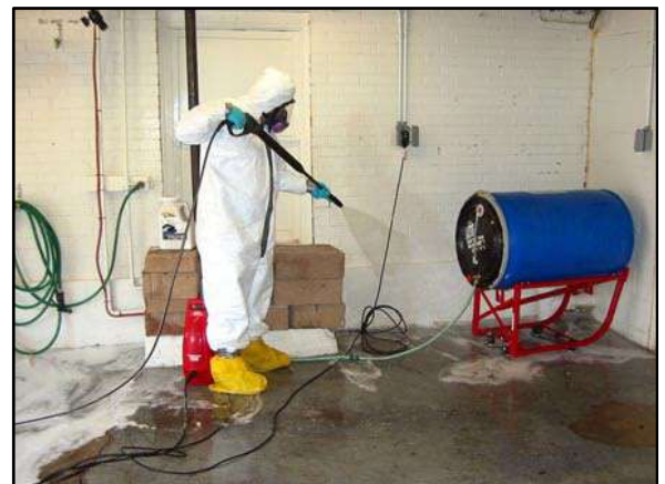
Fig 2. Using a pressure washer to clean contaminated surfaces.
