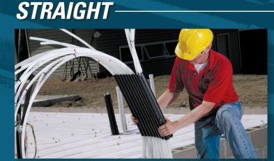
The **Straight** product is an add-on accessory that can be used with the Premier or the Radius, keeping your tubes directed upward and straight. This allows for easy labeling as well as keeping the tubes out of the way of the masons. This will save time, money and hassle.
